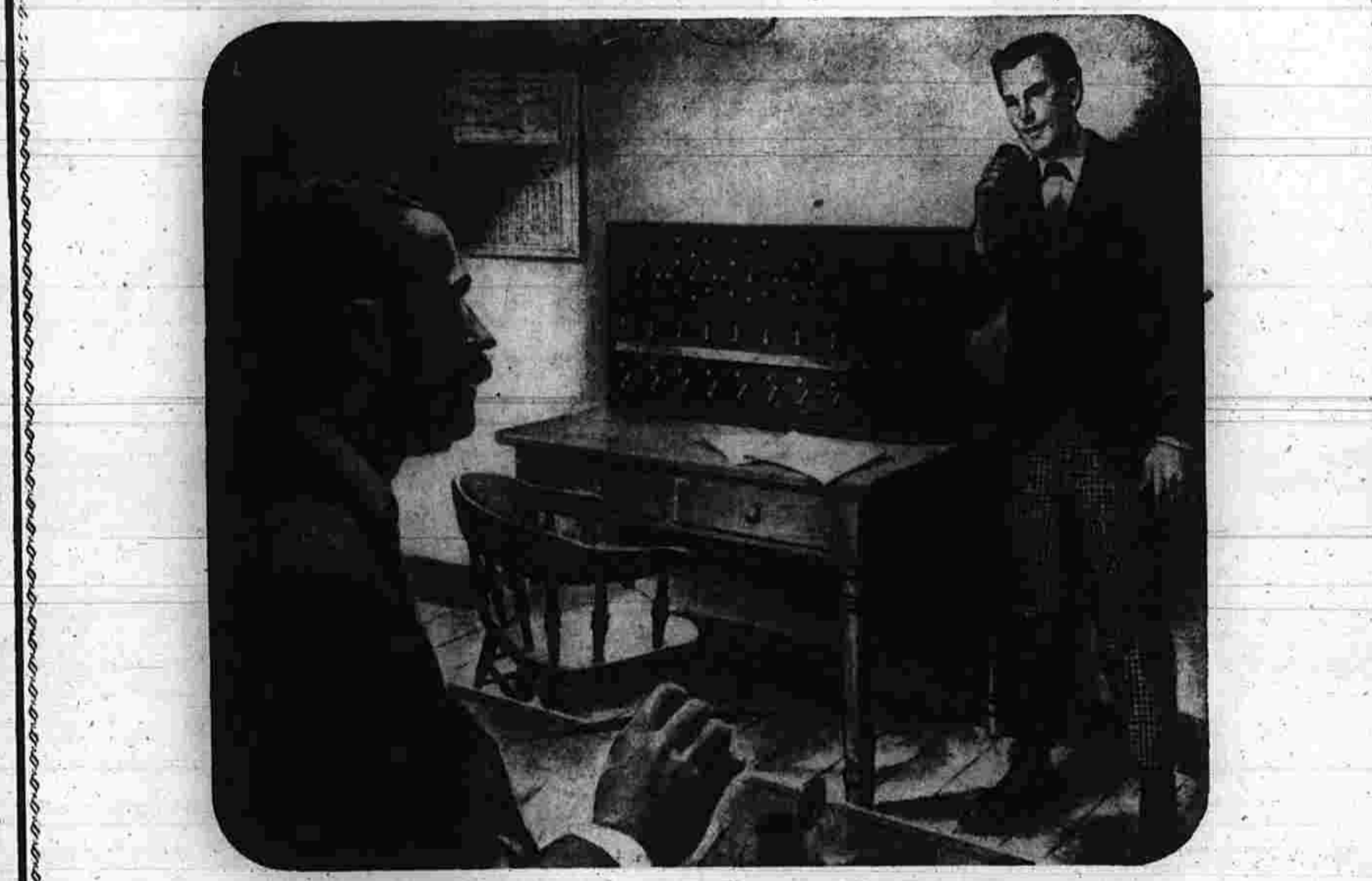
George W. Coy (left) is shown watching boy operator Louis Frost take the first call at the switchboard of the world's first commercial telephone exchange as it opened for business in New Haven, Connecticut, January 28, 1878—75 years ago . . . eight lines, twenty-one subscribers.
